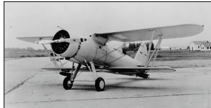
The XF2J-1 fighter at NAS Anacostia on 26 Jun '33, with underwing bombs. Delivered with open cockpits, an enclosed canopy was later added.
